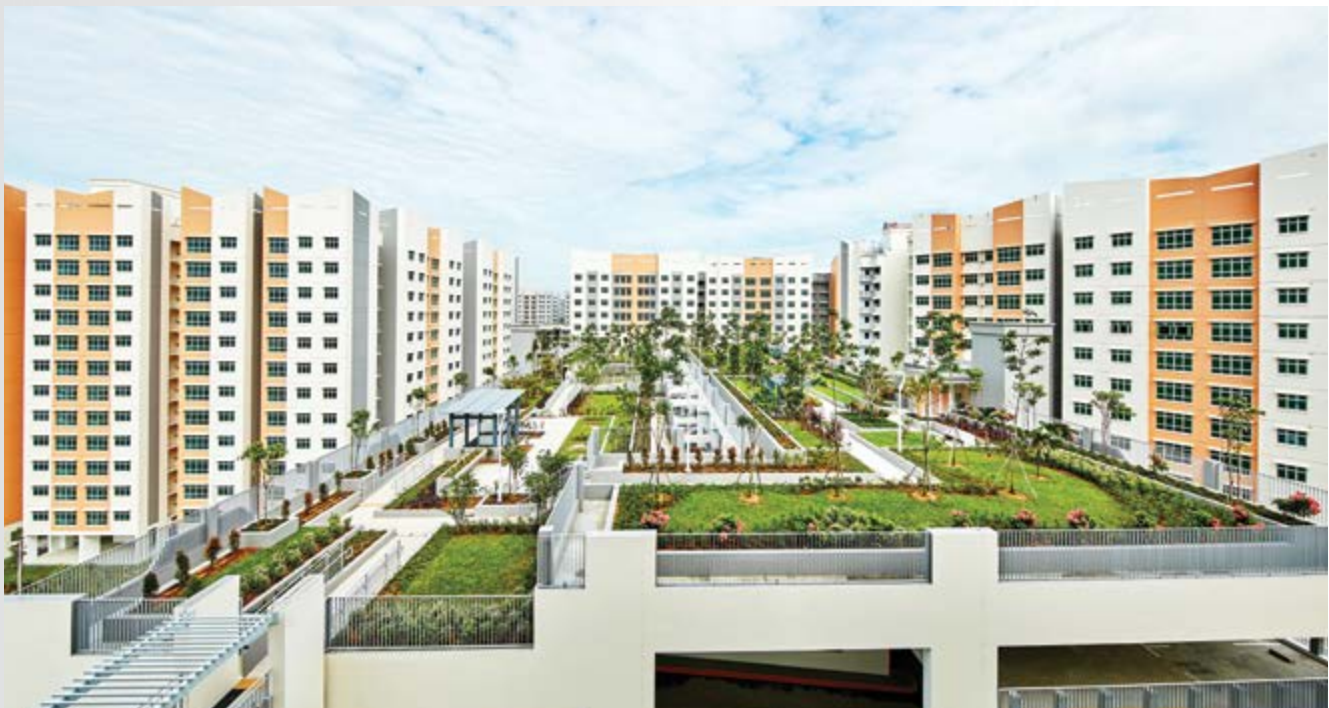
Rooftop Garden @ Sembawang N1C10
