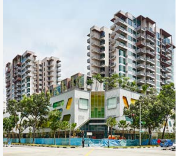
Junction Nine & Nine Residences
